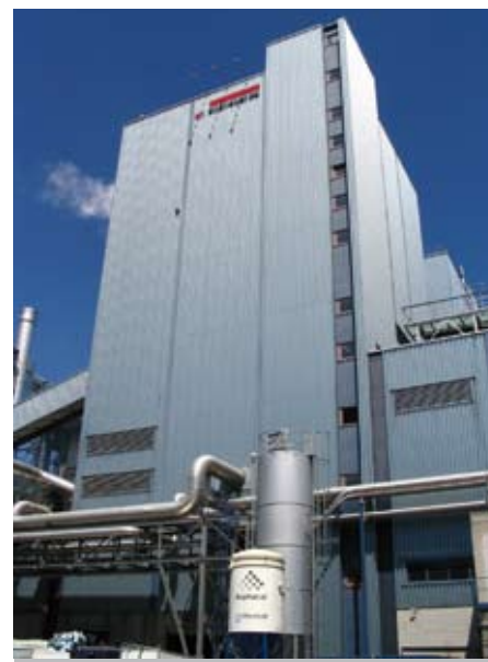
BRILON (DE) , since 1991, extensions 1993 and 1996. Combustion heat generation: 150 MW Steam generation capacity: 165 t/h
