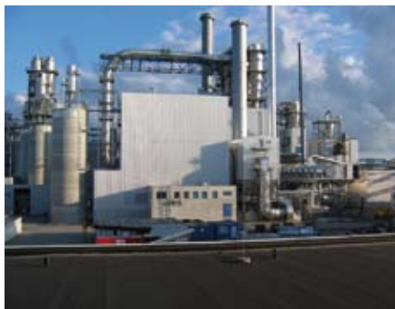
WISMAR (DE) , since 1999, extension 2006. Combustion heat generation: 80 MW Steam generation capacity: 101 t/h
