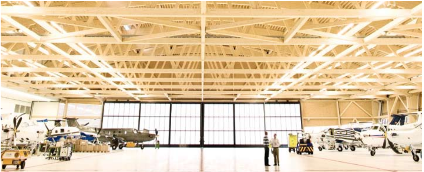
The assembly hall of the Pilatus Aircraft Ltd. in Stans is almost completely constructed of wood. The excellent static and structural-physical characteristics were decisive for the choice of EUROSTRAND® OSB 4 TOP as planking for the load bearing structure.
